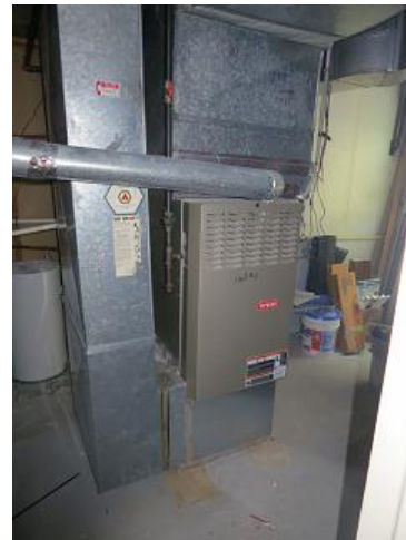
Image 8: Indoor Evaporator with Furnace
