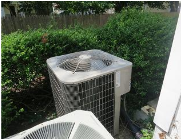
Image 7: Outdoor Condensing Unit
