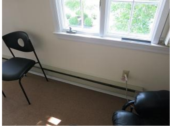
Image 12: Electric Baseboard Heater
