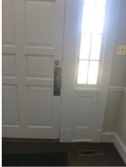
Image 7: Exterior Doors with Gap
