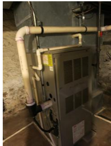
Image 10: Indoor Evaporator and Furnace
