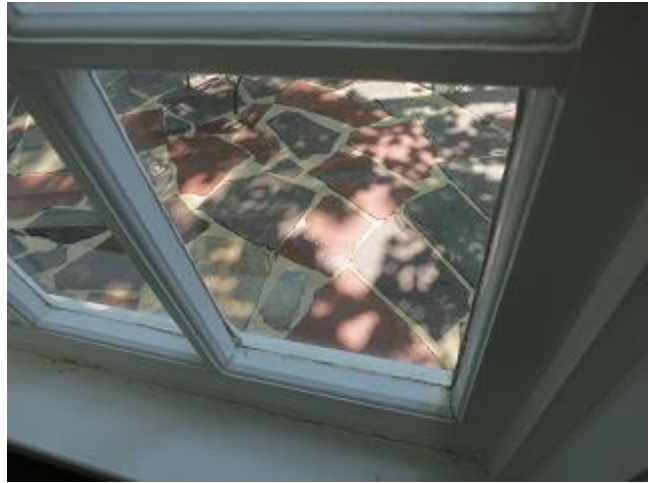
Image 8: Single Pane Window with Wooden Frame
