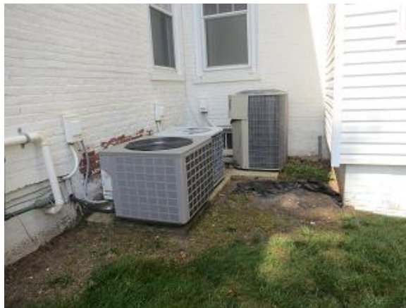
Image 9: Outdoor Condensing Units
