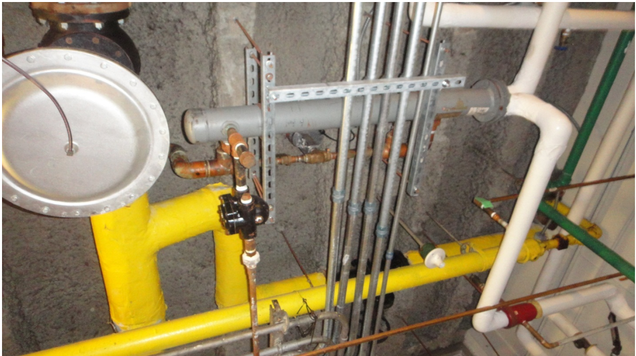
STEAM TO HOT WATER HEAT EXCHANGER
