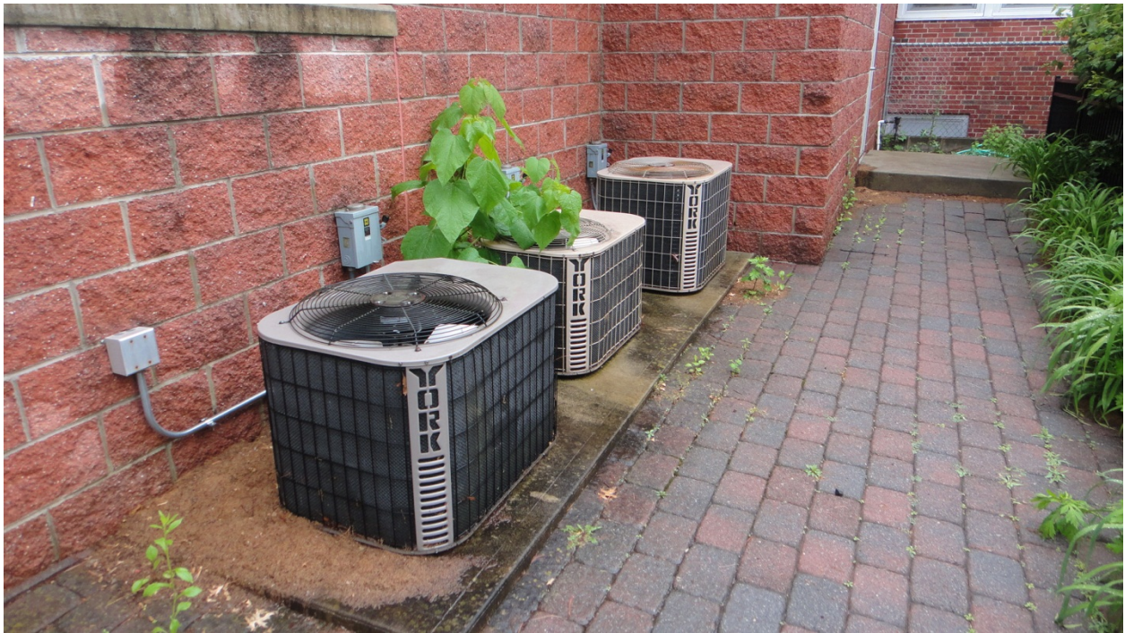
AIR COOLED CONDENSING UNITS ON GRADE
