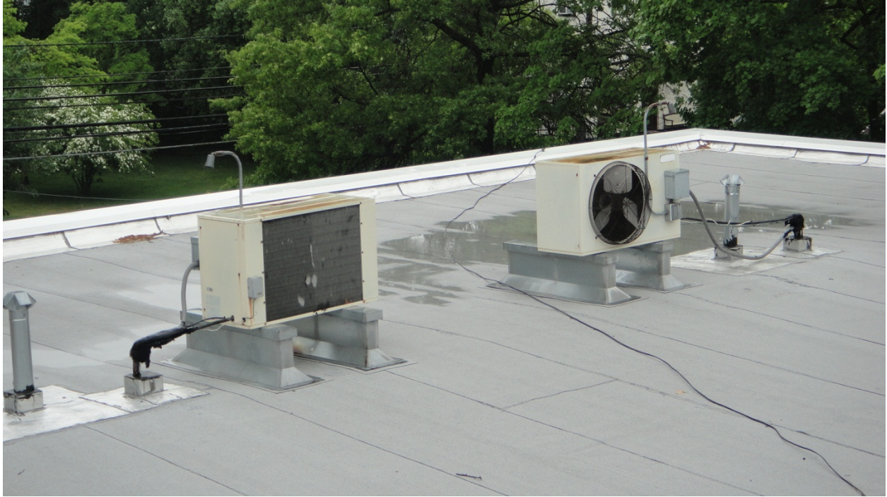
AIR COOLED CONDENSING UNITS ON ROOF
