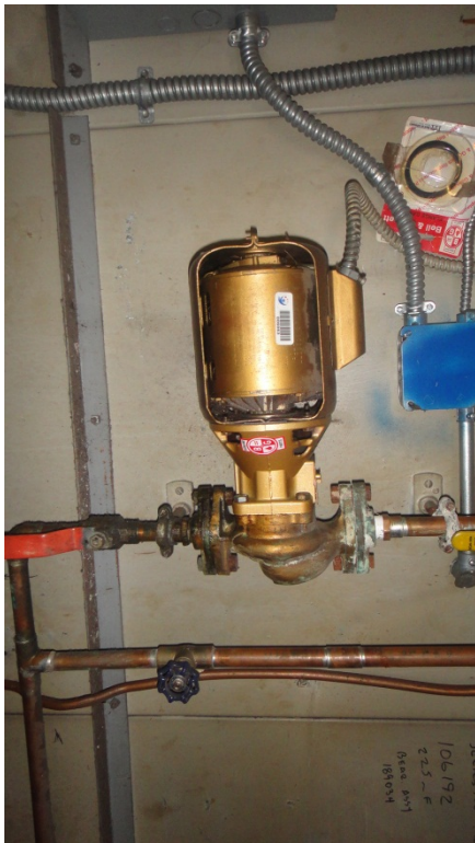
DOMESTIC HOT WATER CIRCULATING PUMP
