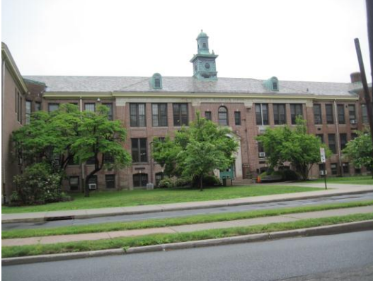
Existing Window ACs
