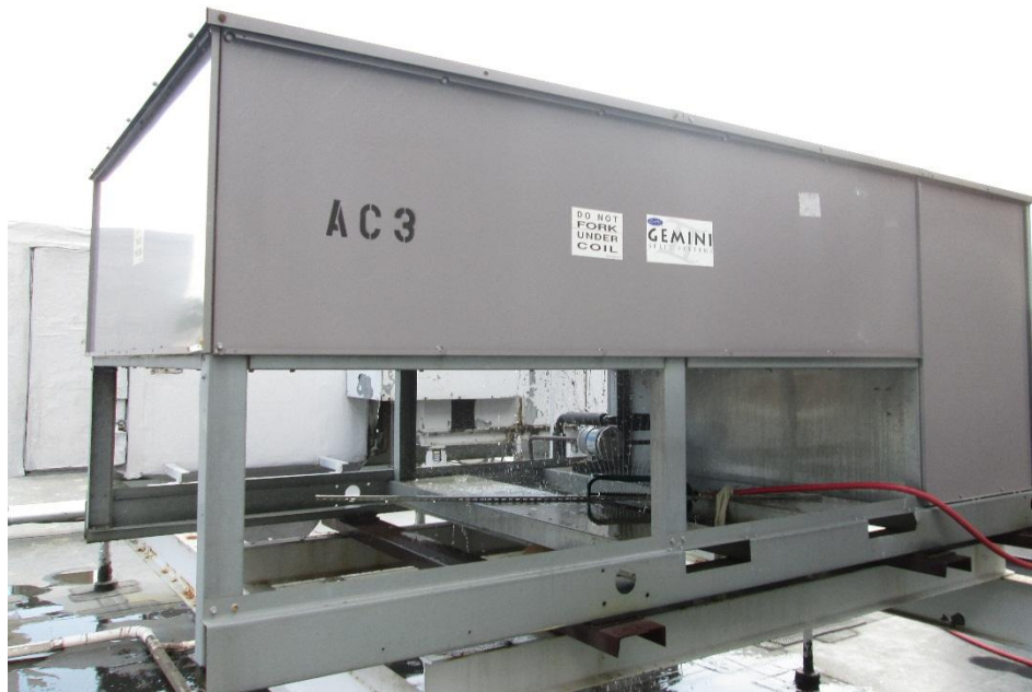
3. Old AC unit with DX coil
