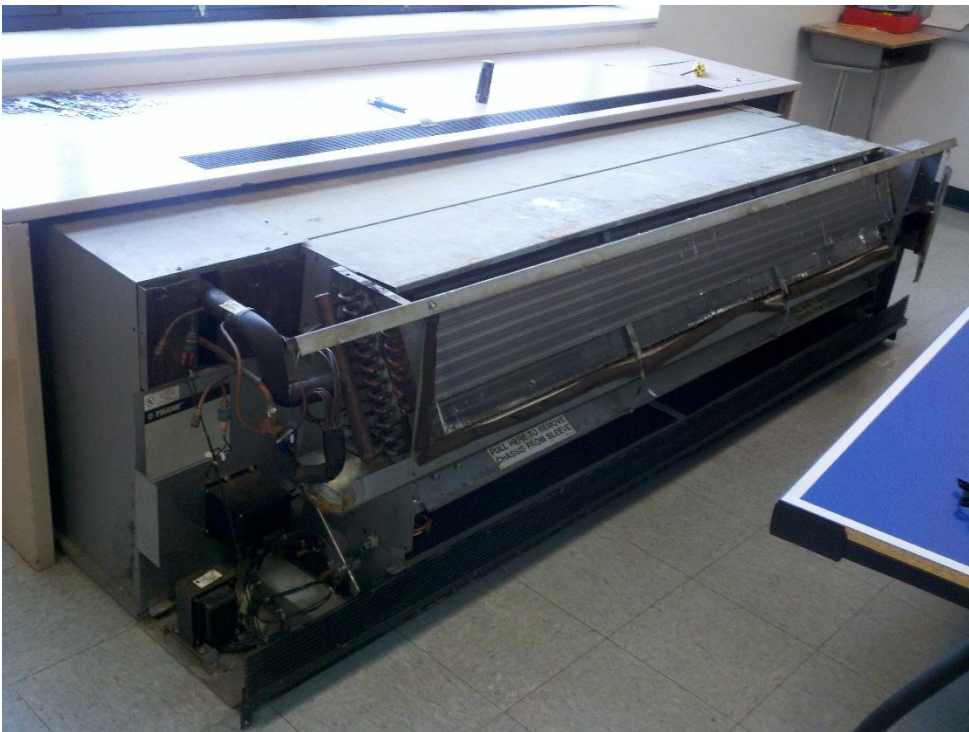
Typical Self-Contained Classroom Unit Ventilator
