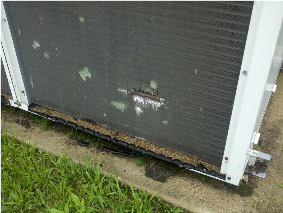
Damage to Condenser Coil
