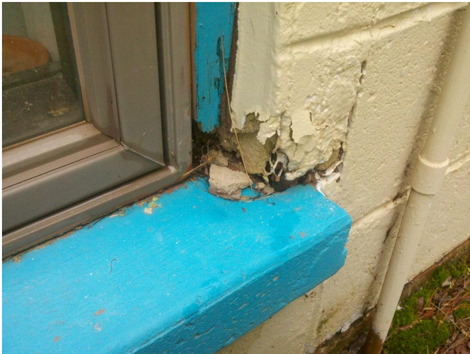
Deteriorated block at window
