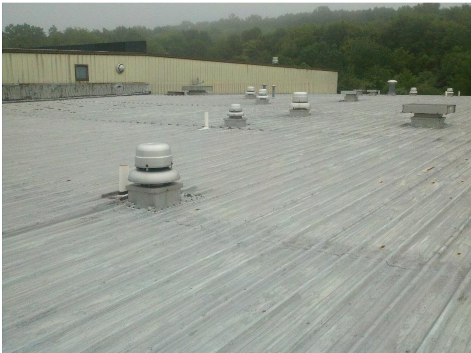
Coated Metal Roof
