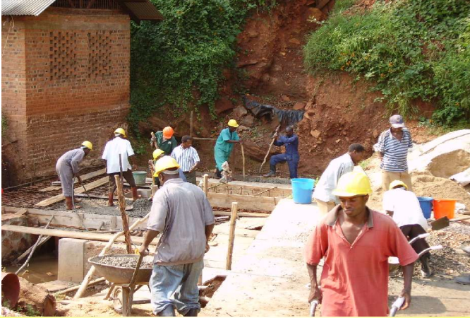
Concrete poured - in one day.
