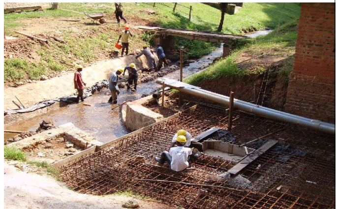
The steel work at the Turbine House, and lined outflow
