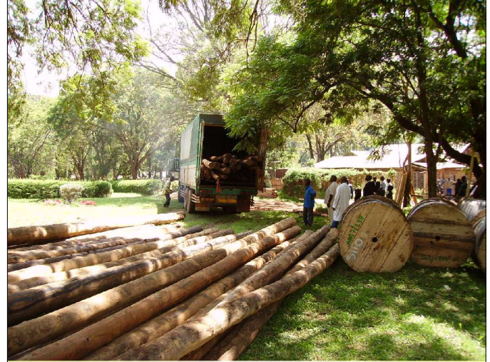
The poles arrive at Kisiizi- and some of the conductor wire.
