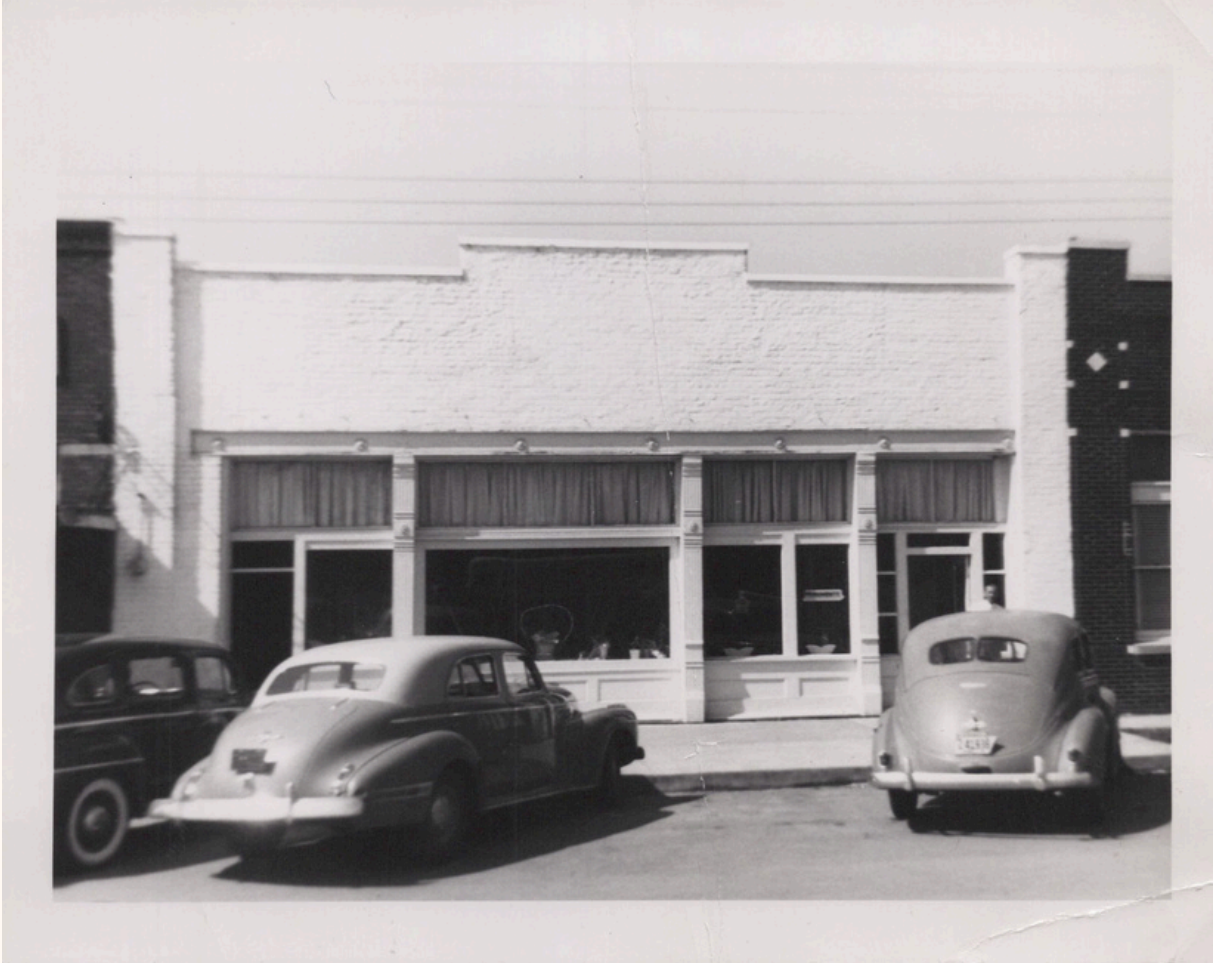
Front Street Location
