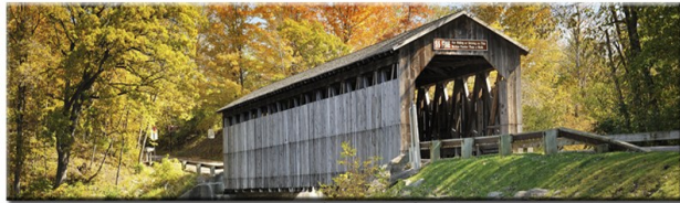
TVC39 - Covered Bridge
