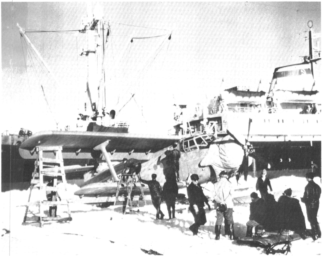
Figure 3. Assembling an AN-2 on fast ice during unloading of Navarin near Amery Base, January 1973.
