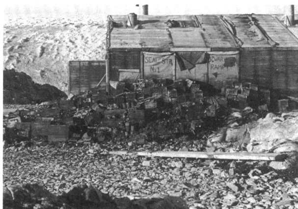
Figure 9. Broken stores and debris piled at the northwest end of the main building. Some of the boxes bear shipping marks identifying them as U.S. Antarctic Service Expedition or individual expedition members’ property. The debris also fills the space between the main and science buildings. The signs were put up by the British who stored dead seals in the main building in recent years. The canvas covering is nearly all gone from the northern parts of the buildings.
