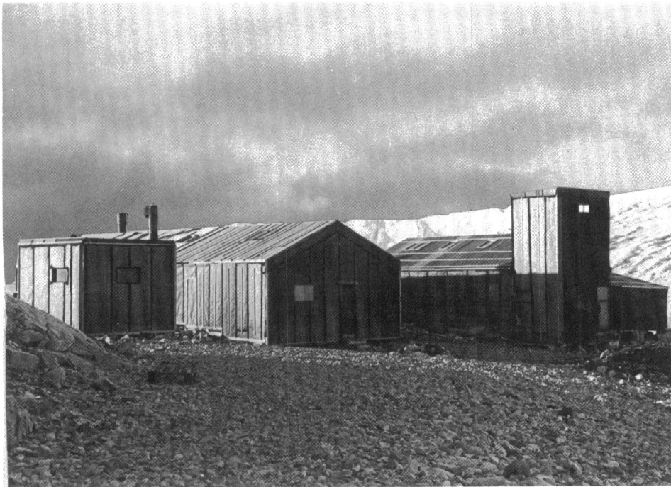
Figure 5. East Base, Stonington Island, showing the southeast side. Left to right: Finn Ronne's hut, the main building, and the science building with the meteorological tower.
