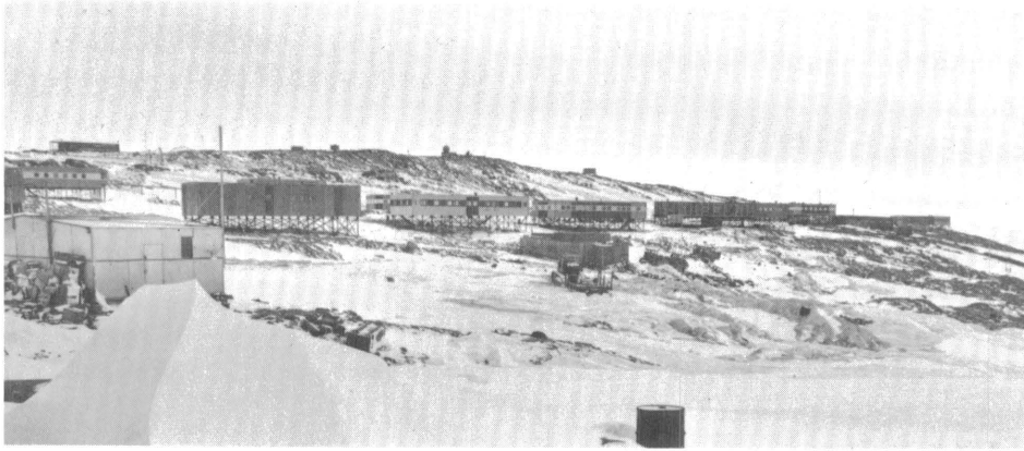
Figure 5. Molodezhnaya Station. Buildings are on stilts to prevent drifting over by snow.
