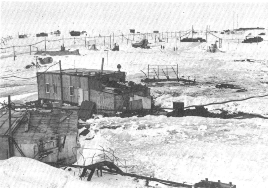
Figure 7. Mirnyy Station. Completed 18 years ago, most of its buildings are drifted over.
