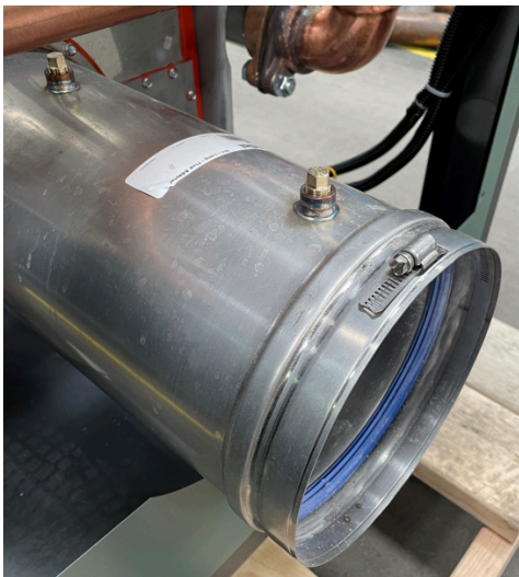
Figure 1. Removal Flue Access Panel
