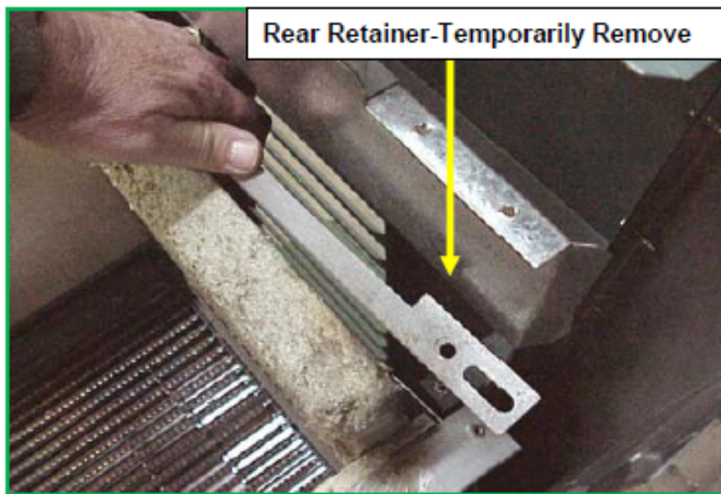
Figure 8. Remove Rear Retainer
