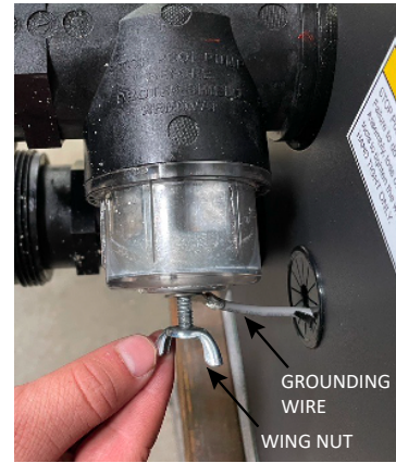
Figure 3. Remove Grounding Wire from ProTek Shield
