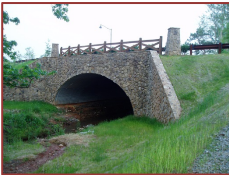
Figure 3-3: Typical Bottomless Arch Culvert w/Headwall
