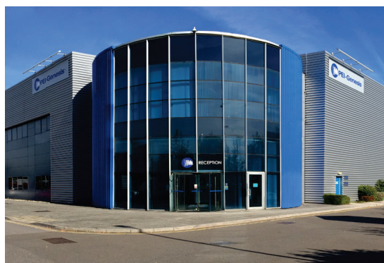
European Headquarters & Production Facility, Southampton, UK
