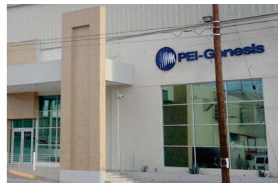
Production Facility, Nogales, MX
