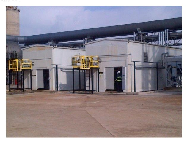
Typical compressor enclosures manufactured by GCL with removable roofs. Less than 80 dB(A) outside with 100 dB(A) inside @ 1m FFC.
