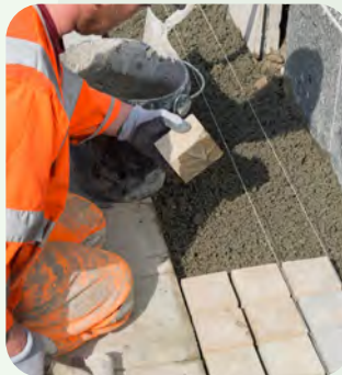
Step 9 Tap unit down to level
