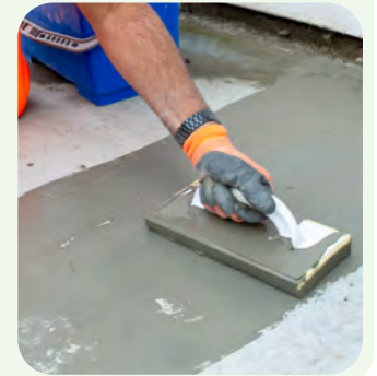
Step 6 Apply bonding mortar to base
