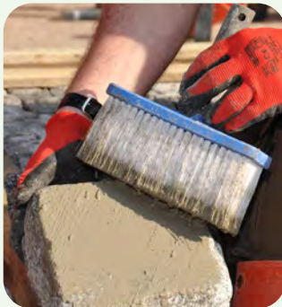
Step 8 Brush on the bonding mortar
