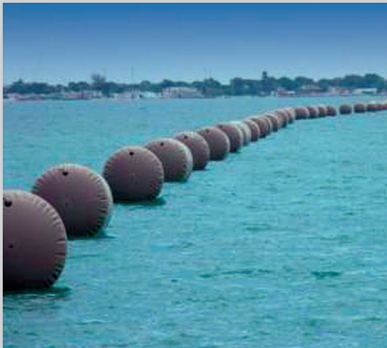
SP-6000's used to support a pipeline during installation.
