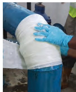
INSTANT LIVE LEAK PIPELINE REPAIR
