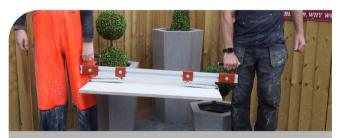
Slab lifters help move flags around safely. Two-man slab lifters are ideal for those heavier flags. The two man slab lifters can be used in pairs for even safer lifting of large slabs.
