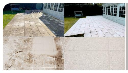
The left-hand photos show the 'before' pictures which illustrate how there can be a haze over the tiles after installation. The right-hand picture shows the tiles after cleaning, as they should be.
