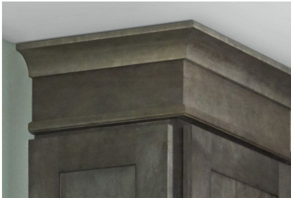
Simple Small Cove Moulding with Single Bead Edge Moulding
