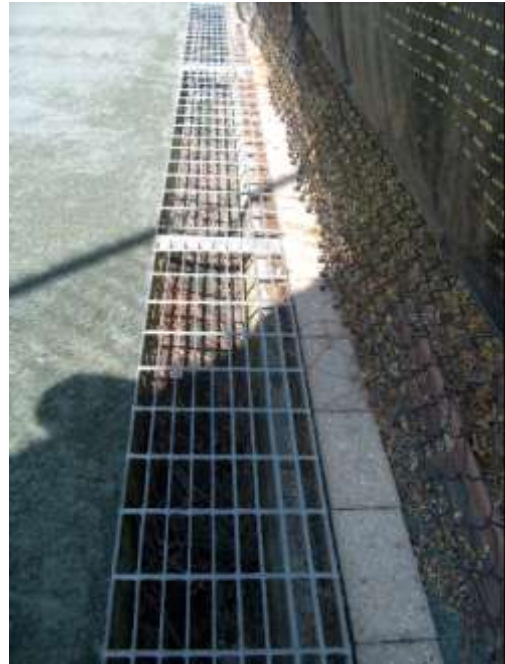
Picture 20 Court Curbing
