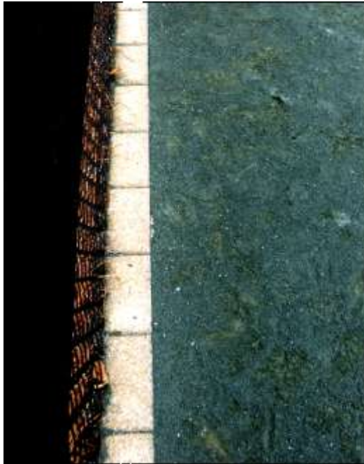
Picture 19 Court Curbing
