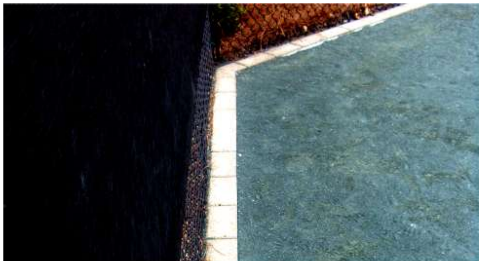
Picture 21 Court Curbing
