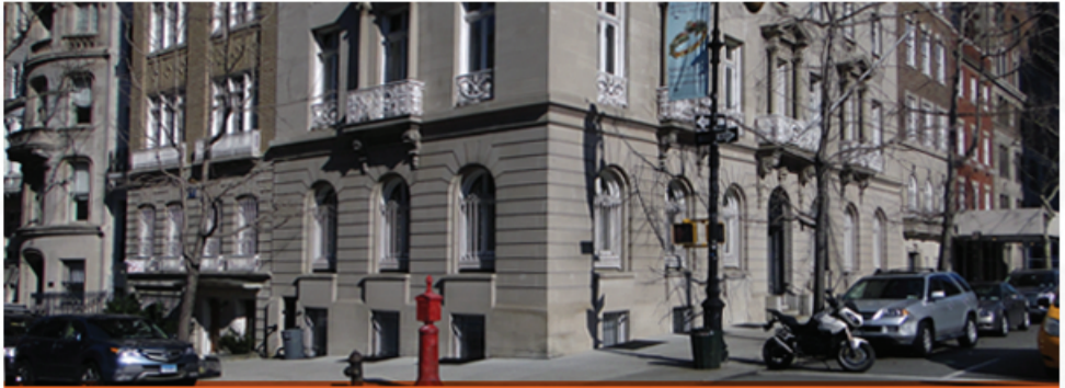
The settled southeast corner
