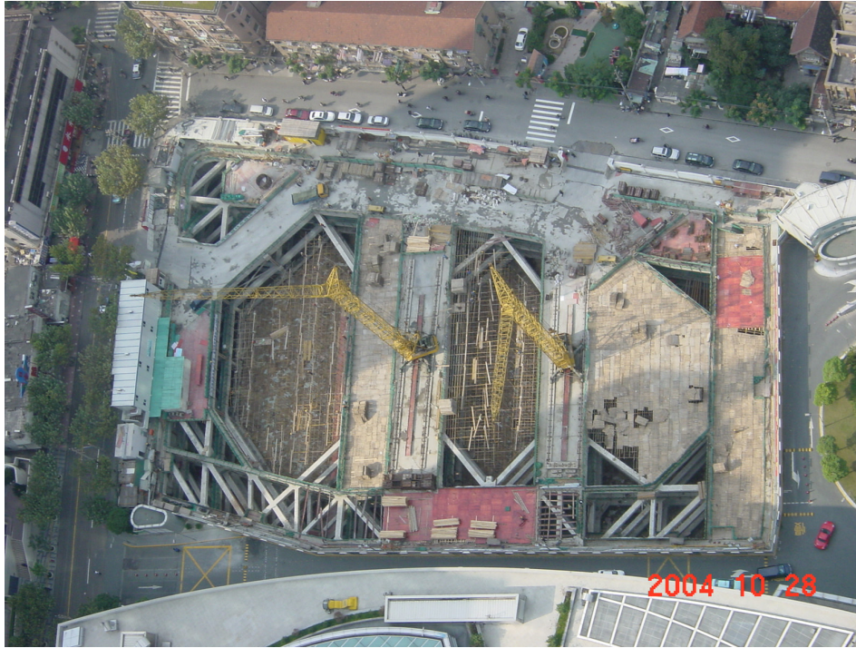
FIGURE 4b - BASEMENT CONSTRUCTION SITE
