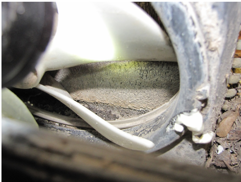
Figure 32. Fouling on the condenser coil of a window AC
