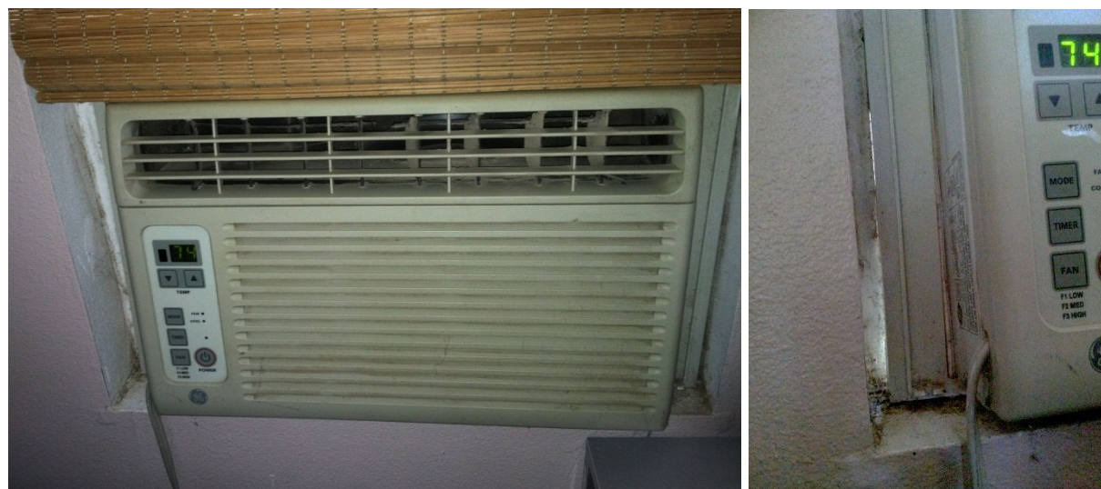
Figure 28. Window AC before retrofit (right). Left view shows a portion of the area where installation air sealing was unsuccessful. The cobwebs, moisture damage, and dirt are further indications of long-term airflow.
