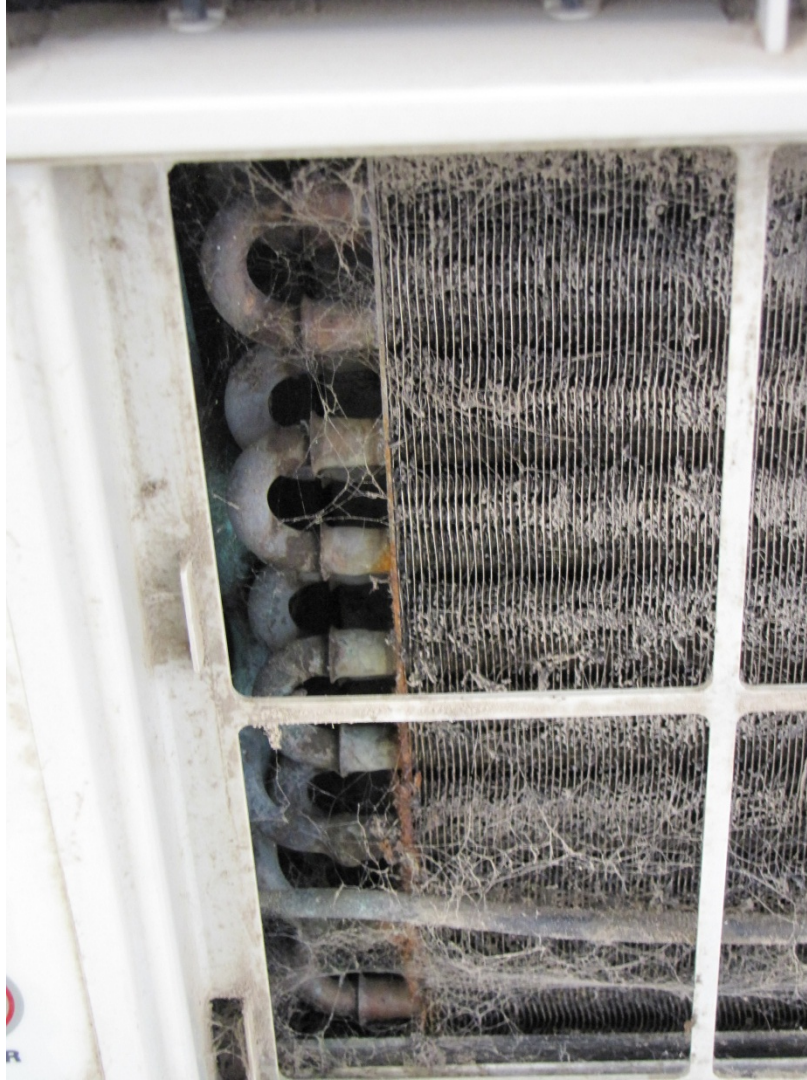
Figure 31. Fouling on the evaporator coil of a window AC
