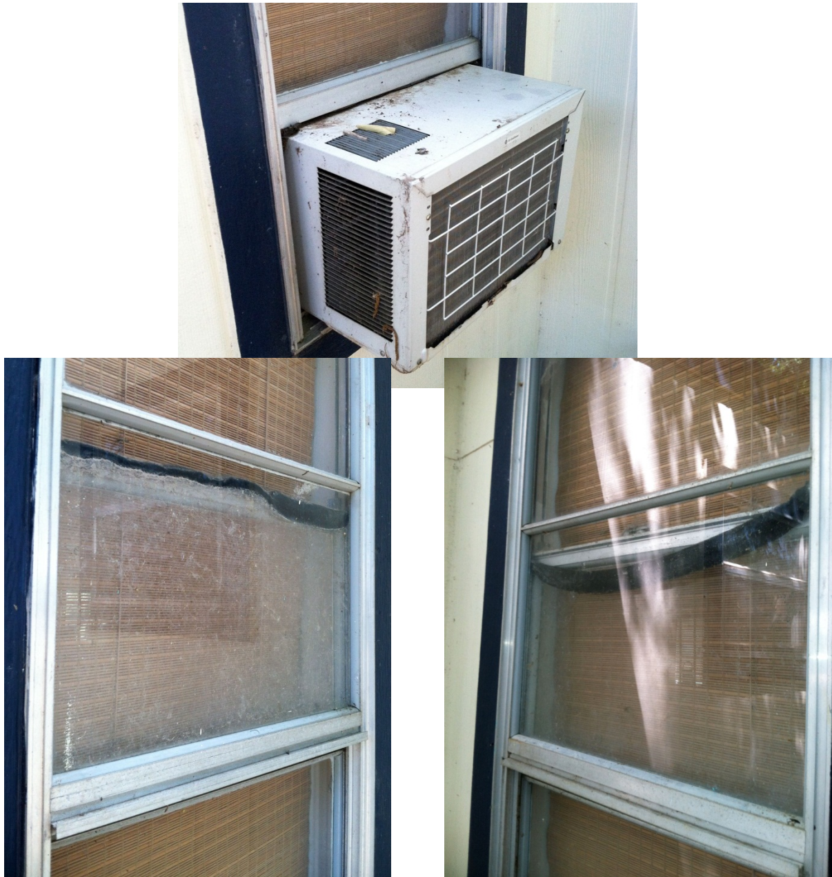
Figure 29. Window AC from the home's exterior (top). Bottom left image shows the window above the tested unit, with foam strip in place between window panes to block airflow. The foam acted as an air filter and did not block air, as indicated by the roughly 12 months of buildup between the otherwise clean window panes. Bottom right image shows the window above the other GE window AC, with the same foam strip installed incorrectly and failing to filter or block appreciable airflow.
