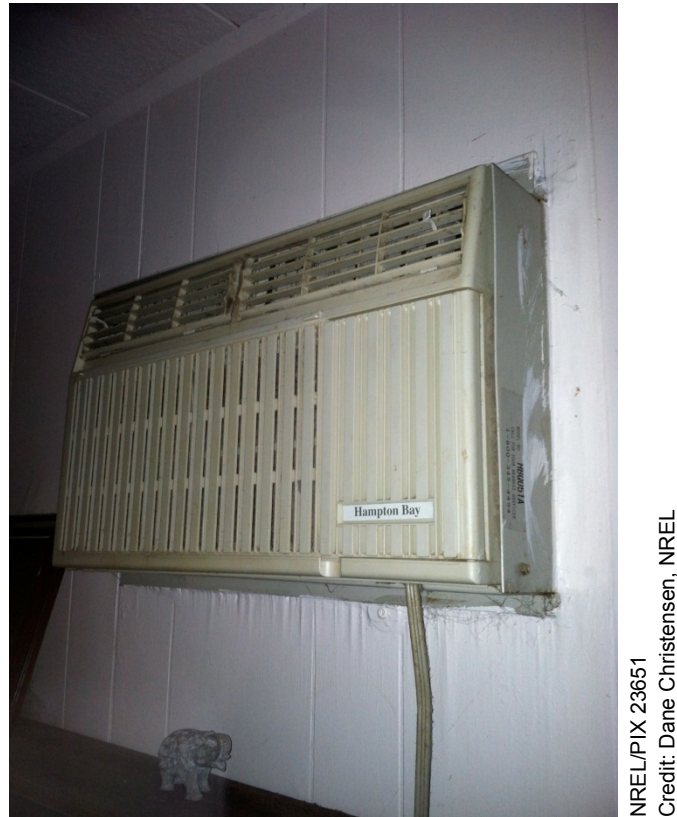
Figure 30. Wall AC showing infiltration- and condensate-caused water damage to interior paneling
