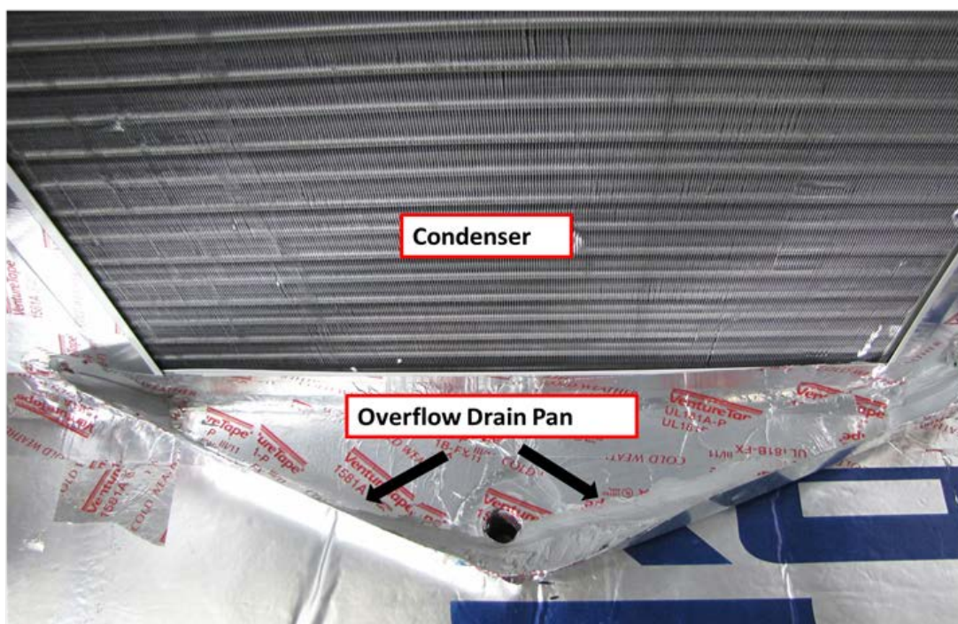
Figure 18. The condenser overflow pan and drain
