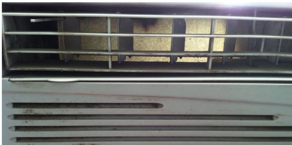
Figure 33. Daylight shining through a window AC firewall. We were unable to locate a fresh air damper, which is a feature of some window ACs and may have provided the opening for this light, which indicates the presence of a large hole, and thus air infiltration.
