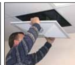
Ceiling speaker array also installs in standard ceiling grid
