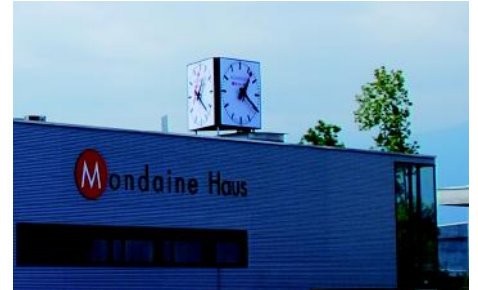
Mondaine production facilities & distribution hub in Biberist/Solothurn
