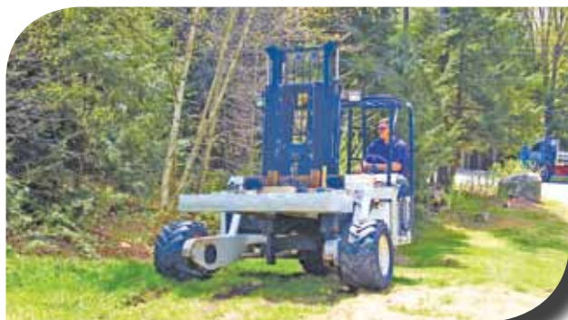
STEP 1: Steps are installed using an all terrain forklift.
