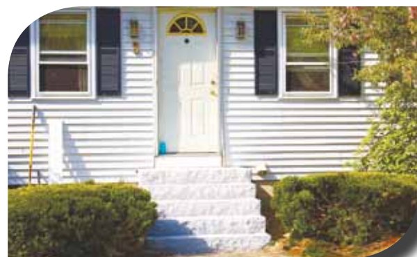
STEP 5: Completed stair case, all that is needed now is a little landscaping!
