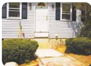
STEP 2: A cement pad is required on all step installs.
