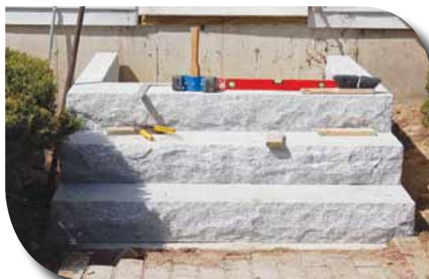
STEP 4: The granite is dry laid, the weight of the steps keeps everything in place.
