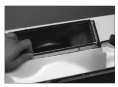
5. Mount starting collar (provided) at rear discharge opening with gasket.
