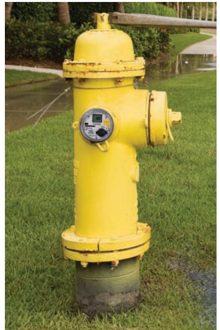
Fire hydrant adapter (A793) necessary to connect to fire hydrants.
