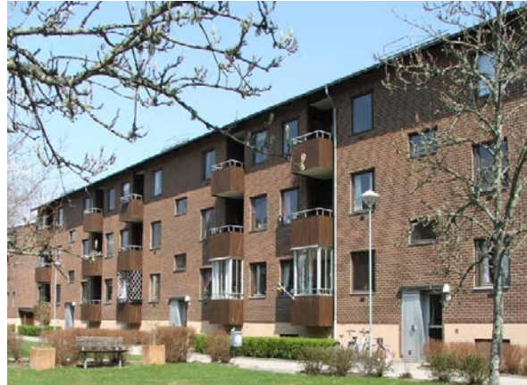
Analysed building in Ronneby
