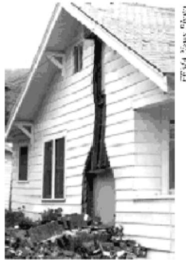
Figure 4 - Northridge Earthquake, Jan. 17, 1994 Chimney Collapse - common type of damage to unreinforced masonry.
