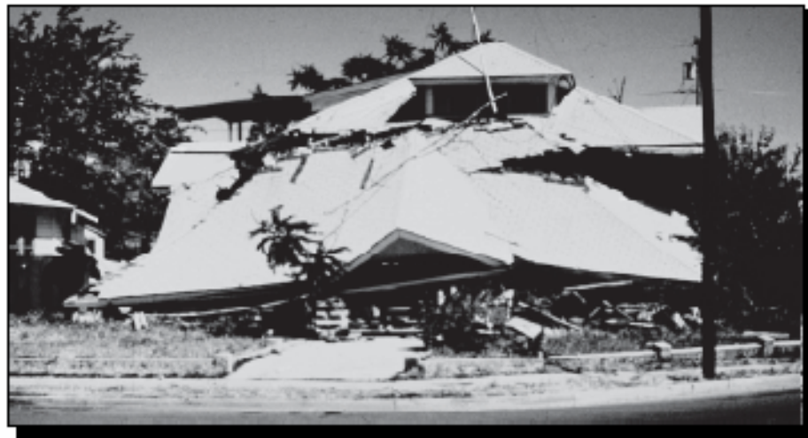
Additional damage from aftershocks
