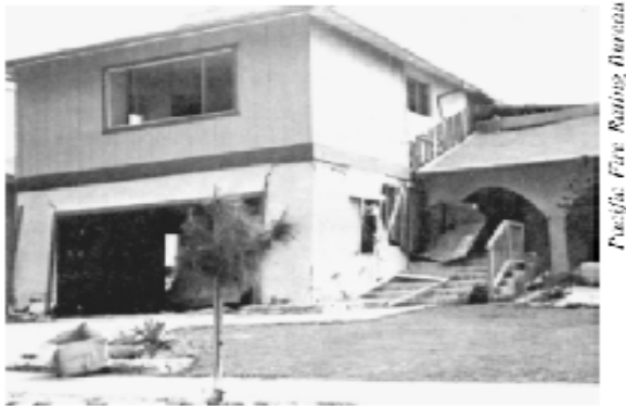
Figure 1 - San Fernando Earthquake, Feb. 9, 1971 Severely damaged split level 1 and 2 story wood frame dwelling. The one story portion dropped about 3 feet.
