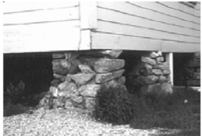
Figure 19 - This is an unreinforced stone foundation. They typically fail during earthquakes.
