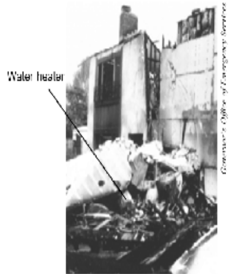
Figure 10 - The unbraced water heater in this home fell during an earthquake; the resulting fire destroyed the home.
