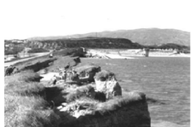
Figure 41 - Lower San Fernando Dam that was badly damaged by the 1971 San Fernando Earthquake.
