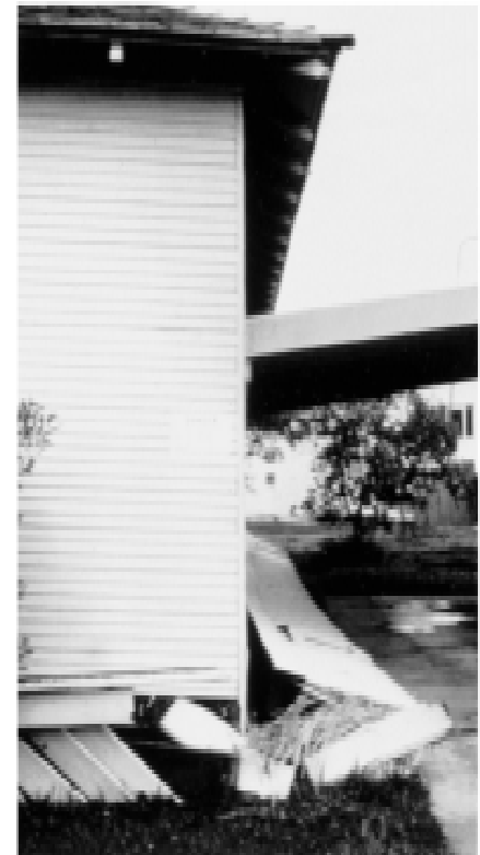
Figure 15 - Damage to home due to cripple wall failure.
