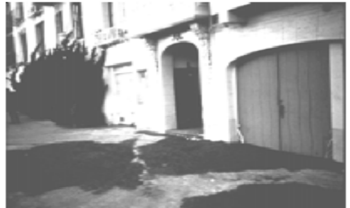
Figure 40 - Loma Prieta Earthquake, October 17, 1989. Lateral spreading, liquefaction and sand boils caused extensive damage in the Marina District of San Francisco, about 60 miles away from the epicenter.
