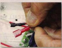
3) We reused the small quick-connect from the Optronics wiring. Star Lights supplies quick-connects, but they are larger.
