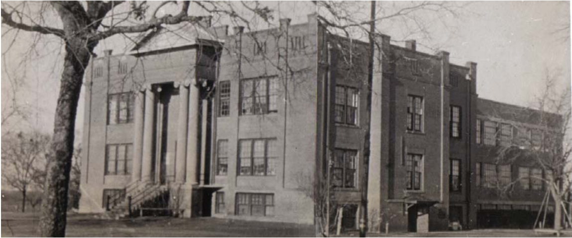
Third Groesbeck School The addition was built in 1922.
