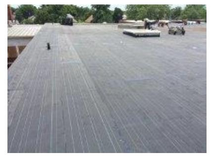
A proper roof expansion joint was installed to prevent splitting of the roof membrane.
