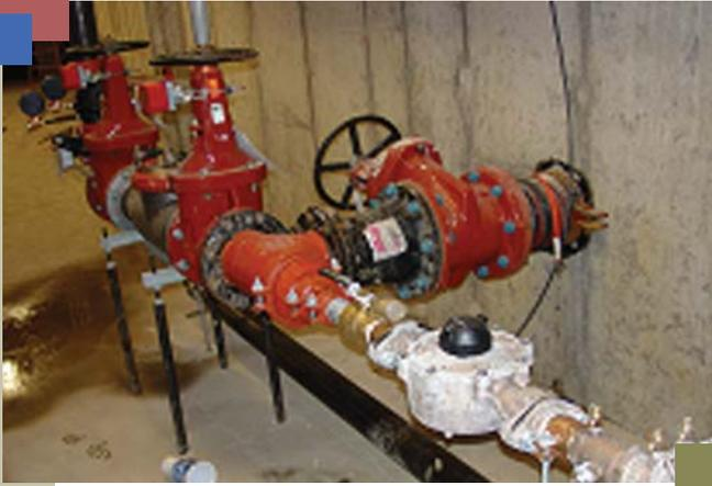
*A building's water supply contains a combination of valves and components to regulate pressure, prevent backflow, and trap large particles, to keep our water safer.*
