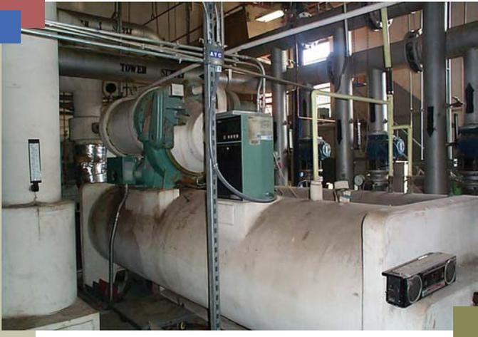
*An air conditioning chiller is a heat exchanger that cools down water. The water is circulated through the building to various cooling coils located in ductwork.*
