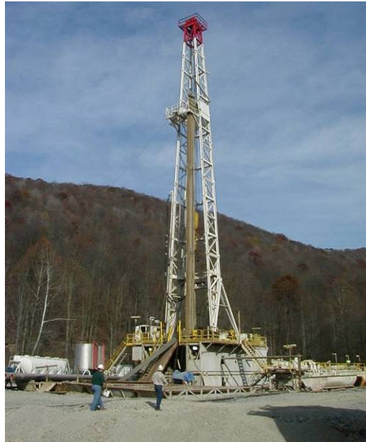
Active Well Drilling – Source: All Consulting
