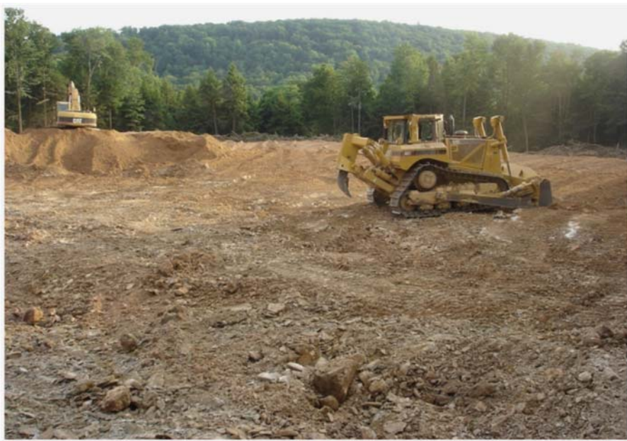
Well Pad Under Preparation (PA) – Source: www.naturalgas.psu.edu
