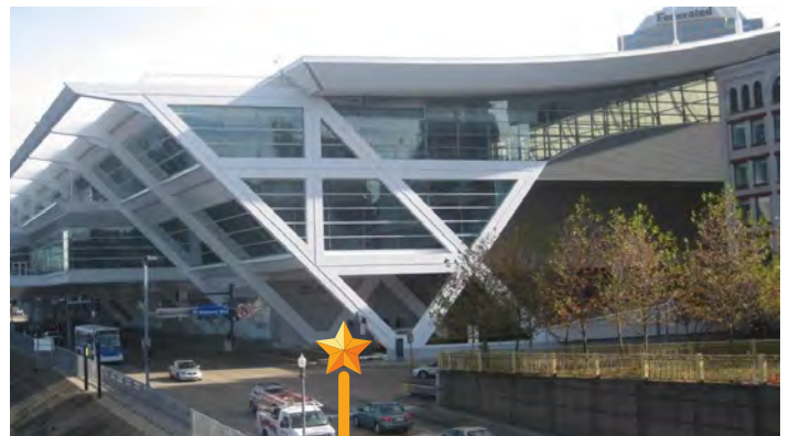
Ft. Duquesne Blvd Loading Dock Entrance
