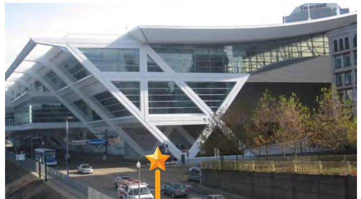
Ft. Duquesne Blvd Loading Dock Entrance
