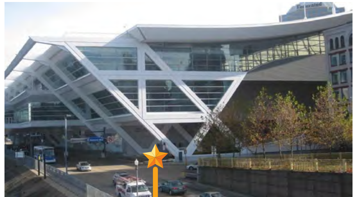
Ft. Duquesne Blvd Loading Dock Entrance
