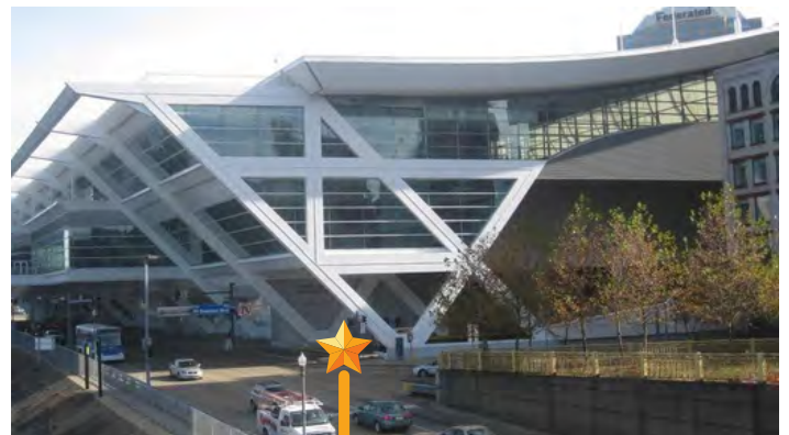
Ft. Duquesne Blvd Loading Dock Entrance
