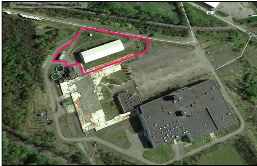
Cortland Industrial Center
