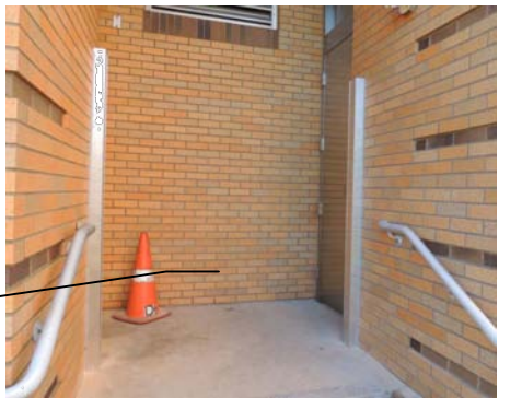
NORTH ENTRANCE WAY STOP LOG RAILS IN PLACE AWAITING DELIVERY OF STOP LOGS ON BACK ORDER
