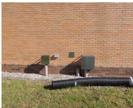
WATERPROOF ELECTRICAL BOXES AND WIRING OR RELOCATE TO ABOVE ELEVATION 15.74
