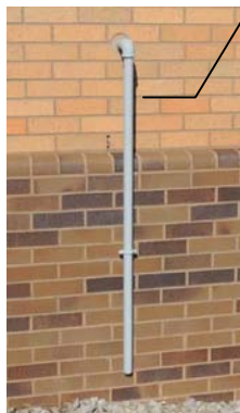
REFURBISH DRAIN WITH VALVE TO CLOSE OFF DURING FLOODING (PENDING)
