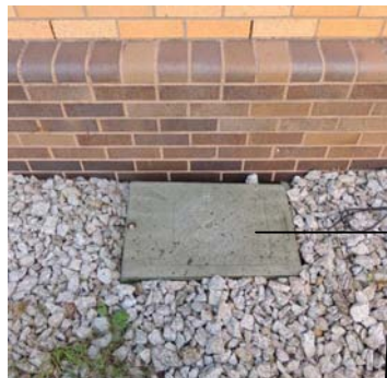
REFURBISH HANDHOLE WITH GASKETED COVER (PENDING)
