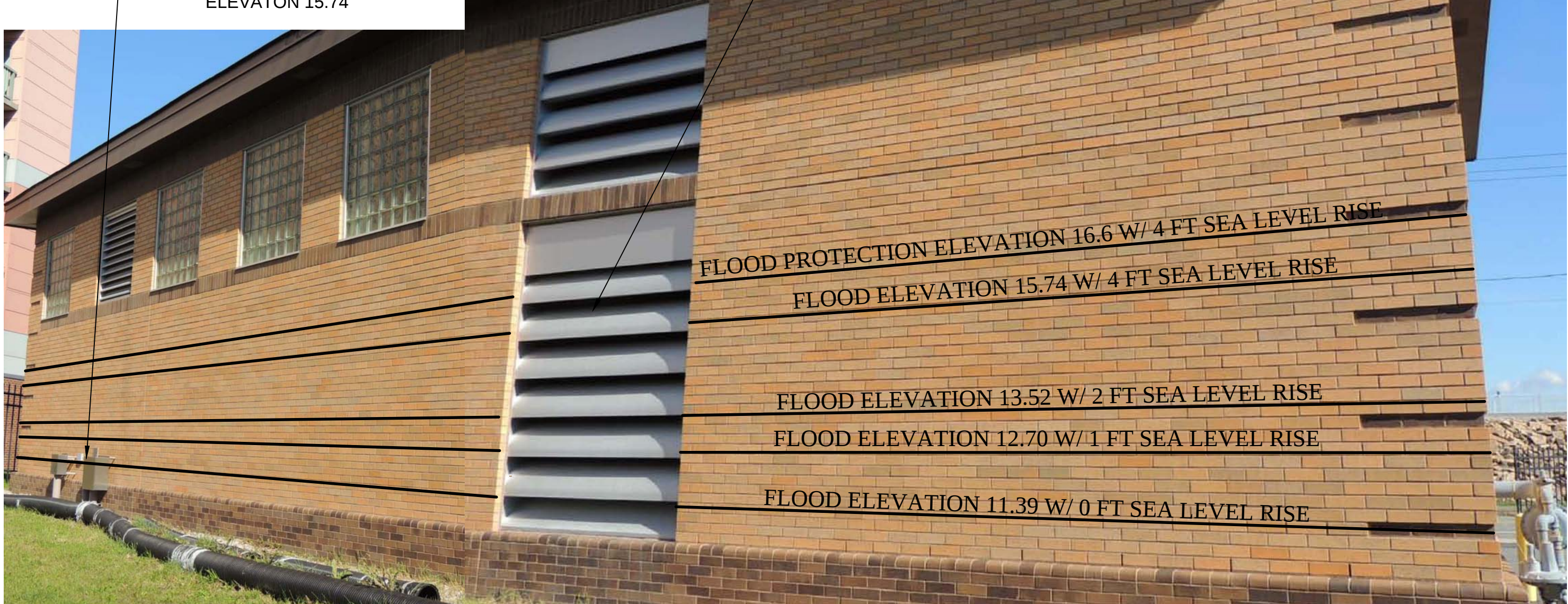
WATERPROOF ELECTRICAL BOXES AND WIRING OR RELOCATE TO ABOVE ELEVATION 15.74
