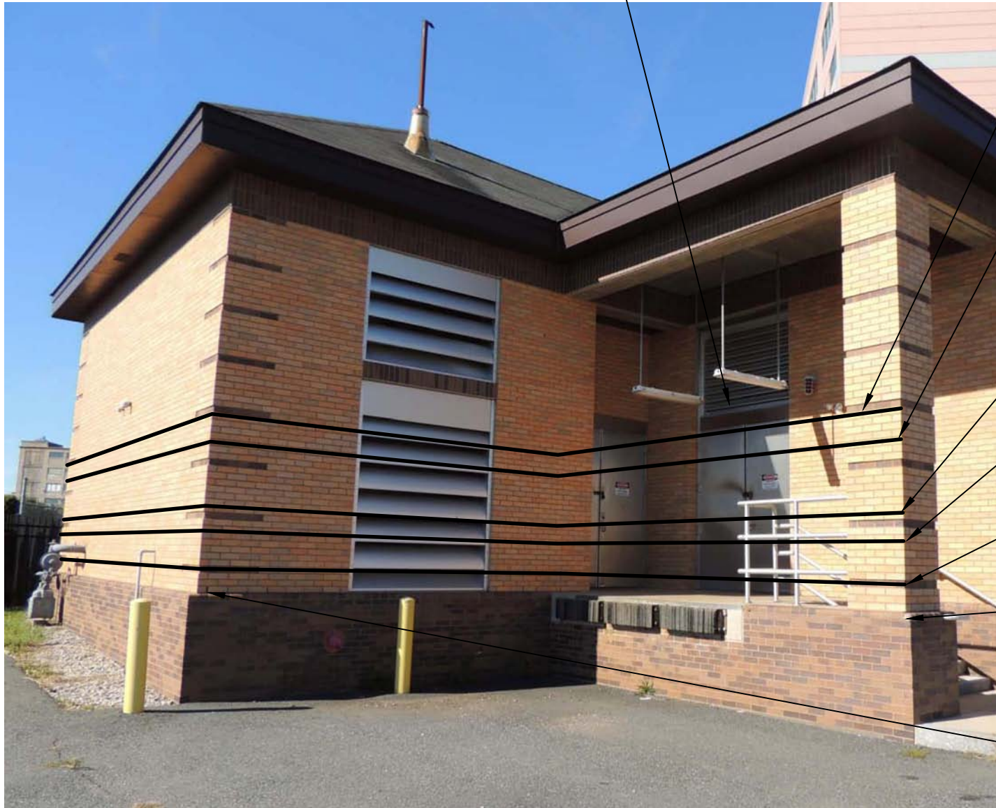
SCREEN ROOM ENTRY DOOR
