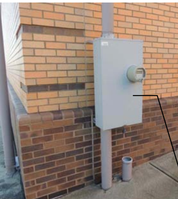
RAISE METER PANEL TO ABOVE ELEVATION 15.74 (PENDING)
