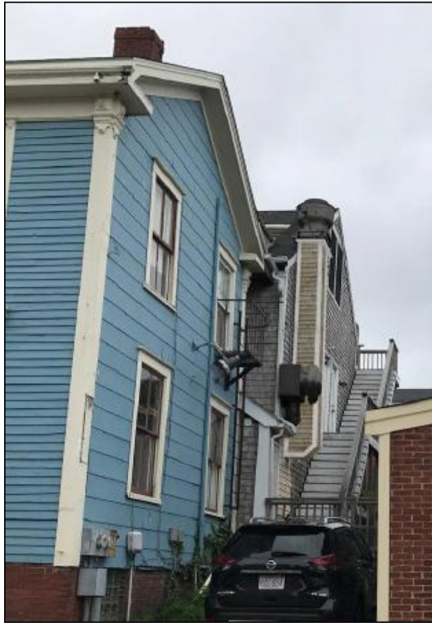
Proposed ductwork screening shaft enclosure with exposed ductwork painted black.
