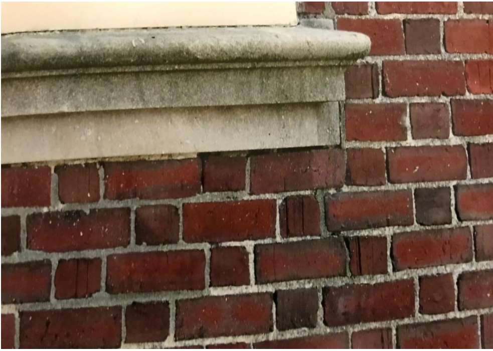
7. Wood Building, North Elevation, deteriorated and cracked mortar and brick
