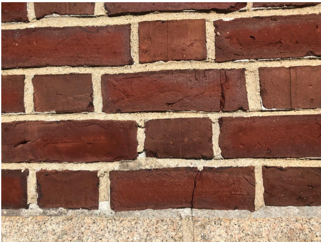
10. Bourne Building, West Elevation, deteriorated mortar, cracked, spalled brick
