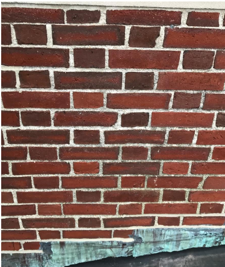
13. Bourne Building, North Elevation, deteriorated mortar, cracked, spalled brick
