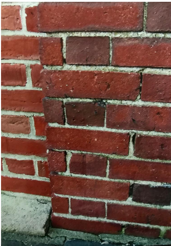
9. Wood Building, West Elevation, deteriorated mortar and brick
