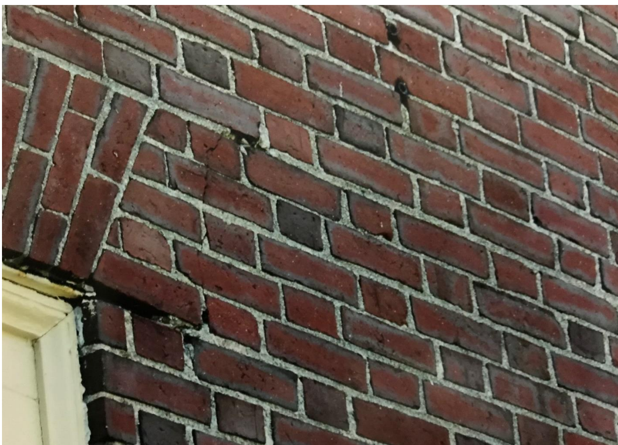
6. Wood Building, North Elevation, failing angle iron lintel
