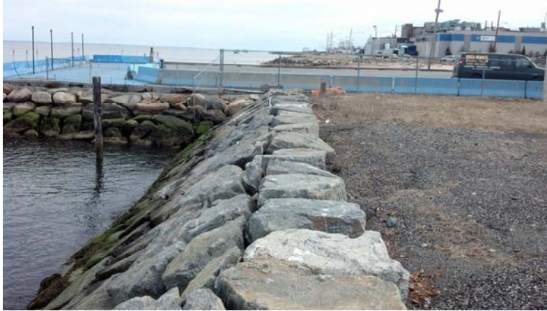
View of existing rip rap shoreline
