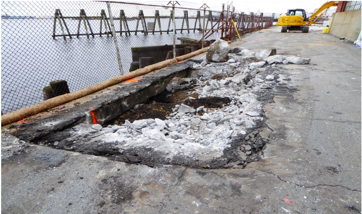
Photo 3: TP-1 prior to excavation, orange markings indicate possible or observed locations of bulkhead support rods. Note thickness of concrete/asphalt layer
