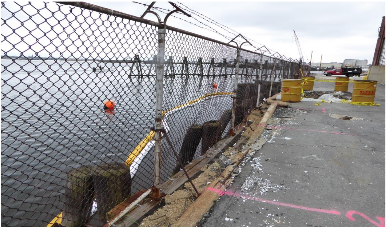
Photo 6 – View of containment and absorbent boom placed in the Acushnet River adjacent to TP-1.
